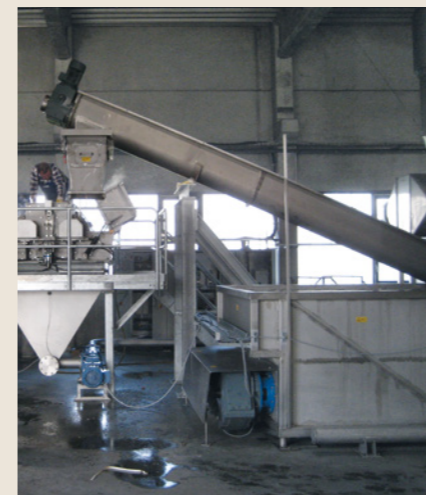
Dosing screw and storage bin (organics)
